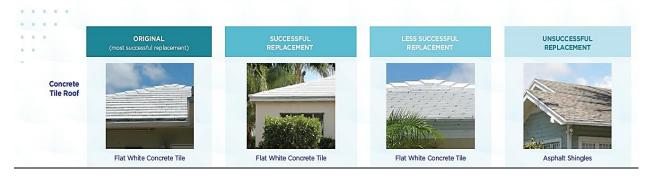
Roof material is an important character-defining feature for a historic property. Per the Design Guidelines, new flat white concrete tiles are the only successful replacement options for original flat white tile roofs. Flat white concrete tiles that replicate historic tile profiles and dimensions are still in production today, and could be utilized as the replacement roofing material.
